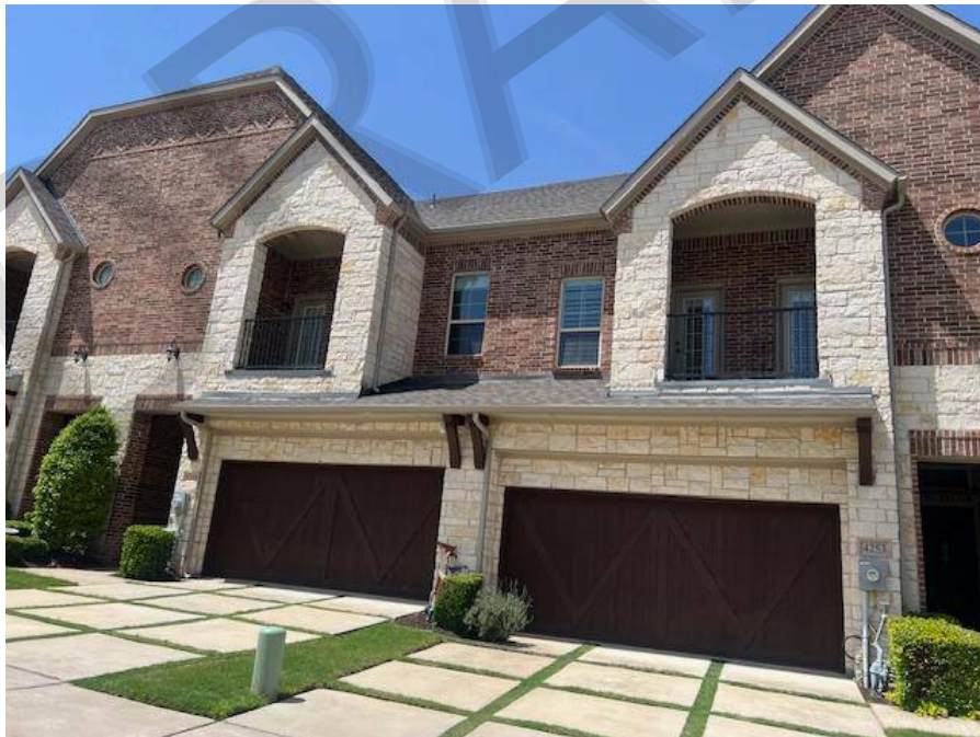
Garage Doors and Exterior Components
