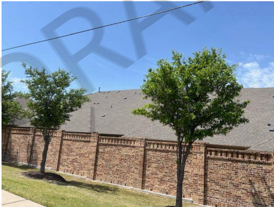
Brick Perimeter Fence
