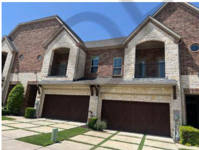
Garage Doors and Exterior Components
